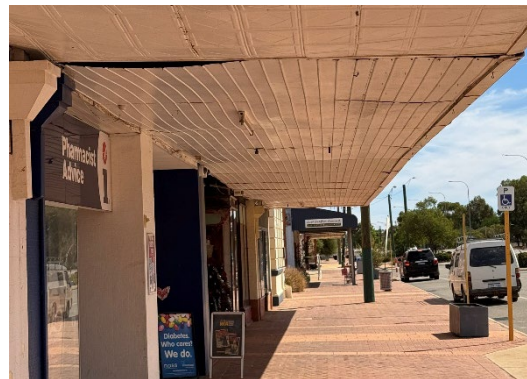
Example of damaged underside of cantilevers.
